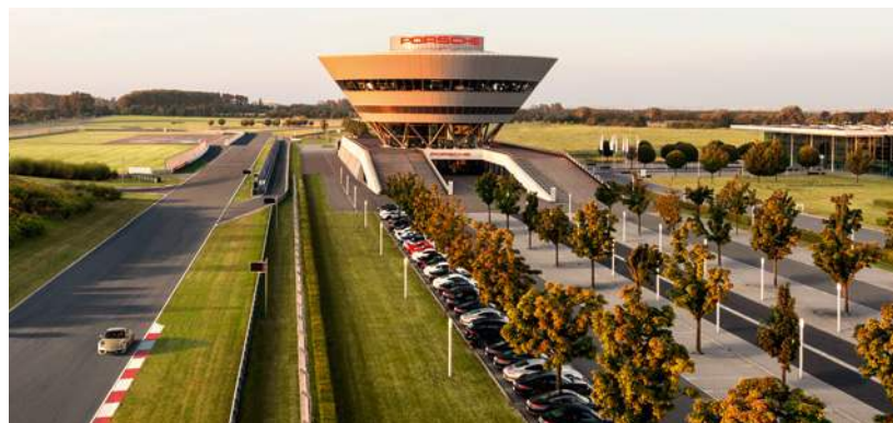
Porsche racetrack and Customer Center in Leipzig
