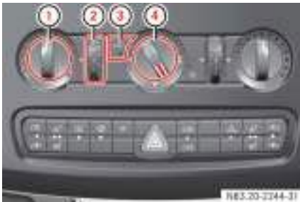
Heater control panel
