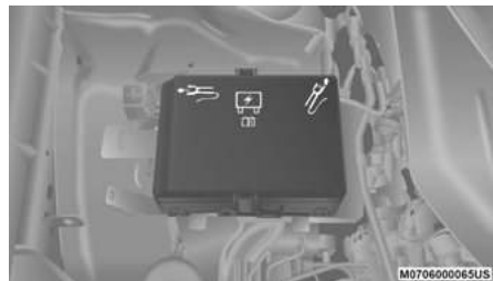
Front Power Distribution Center
