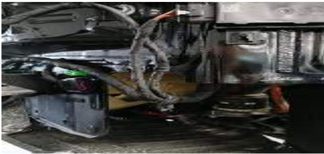
Figure 1: Wiring behind the bumper.
