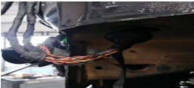
Figure 2: Wiring beneath the wrapping.
