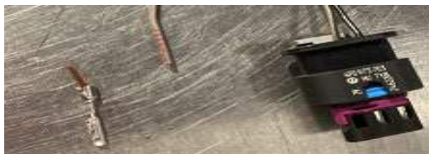
Figure 2: Wire damaged inside G31 connector
