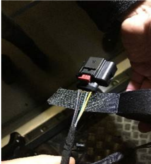
Figure 2. Harness is wrapped using textile tape 105 920 02.
