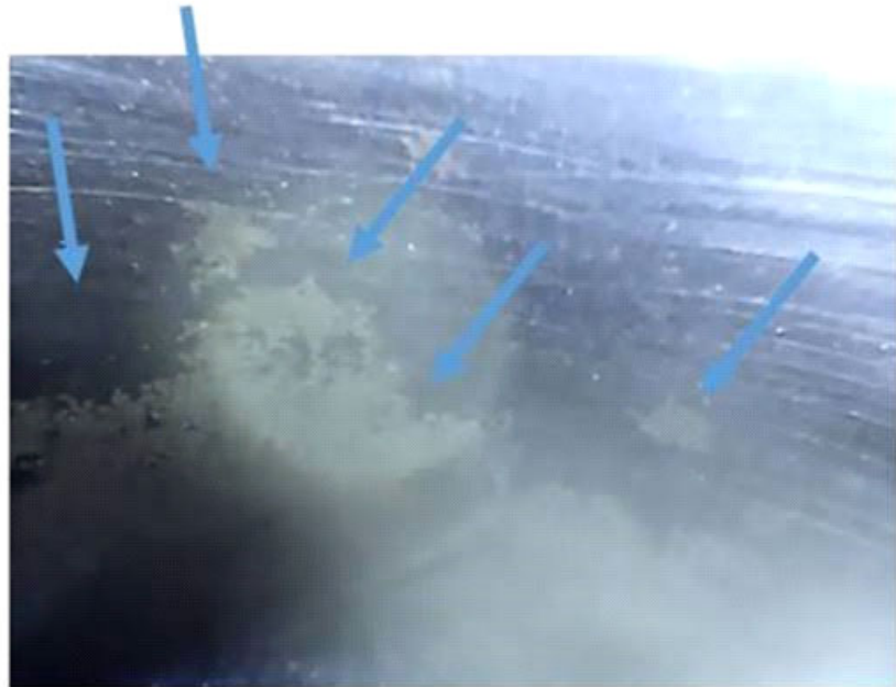
Figure 2. Corrosion marks on cylinder walls (close-up).
