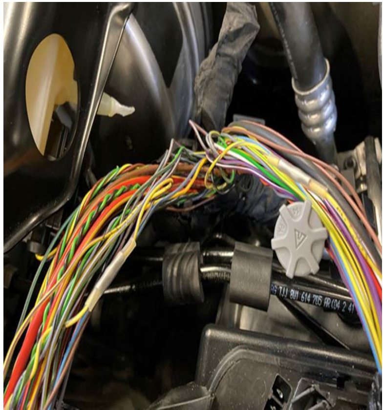
Figure 3: wire modification complete.
