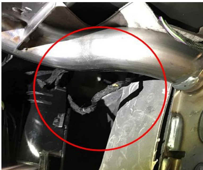
Figure 3: Secure the wires.
