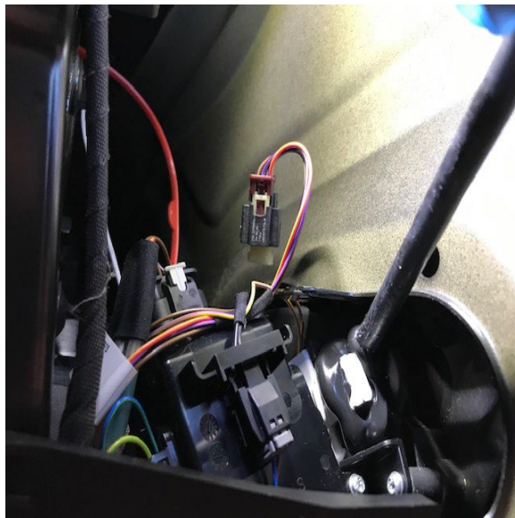
Figure 23: Sealant bead applied at the connector.
