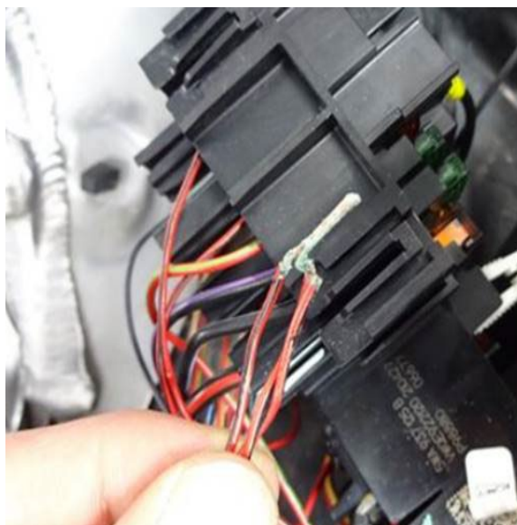
Figure 2: Corrosion found at splice point J1.
