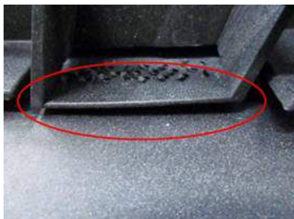
Figure 4. Loose mounting bracket.
