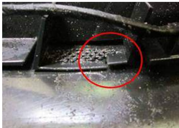
Figure 3. Broken mounting bracket
