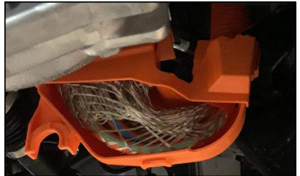
Figure 5. New Part Installed
