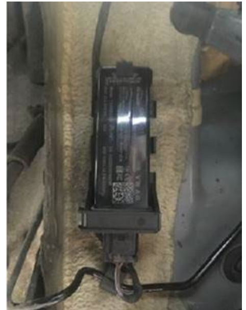
Figure 2. Installation location with new bracket.
