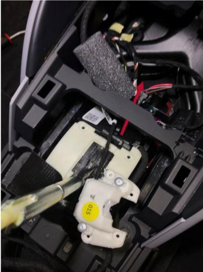
Figure 8. Wiring harness run under the crosspiece.
