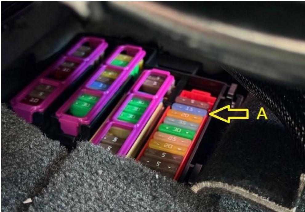
Figure 2. Fuse control panel
