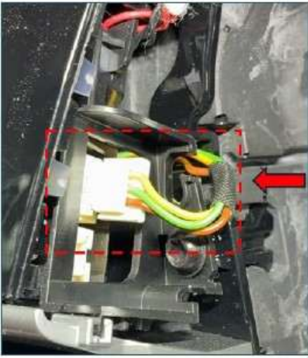
Figure 1. Incorrect wire routing.
