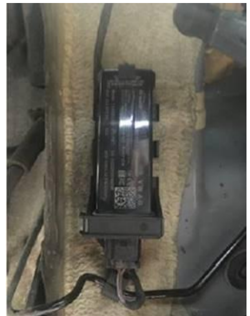
Figure 2. Installation location with new bracket 4E0 810 675 B.
