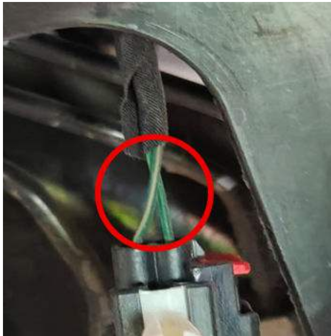
Fig. 5 Area To Inspect For Damaged Wiring
