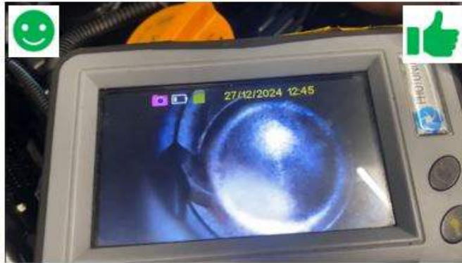
Fig. 4 OK Injector - No Leakage
