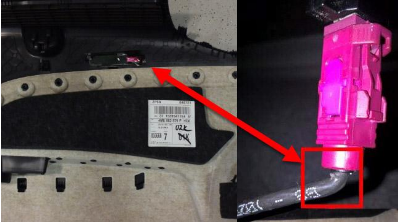
Figure 2. Coaxial wire kinked at R263 SOS Antenna.
