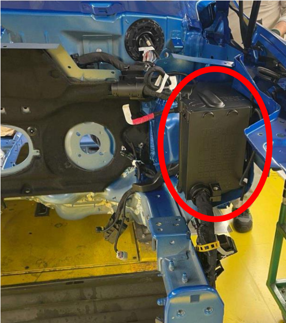
Front Power Distribution Center
